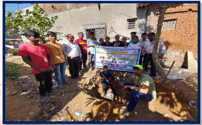
Construction of Soak Pits
